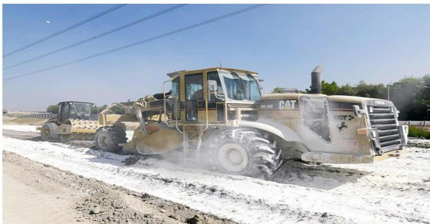
*Figure 1.3 Chemical Stabilization Using Lime*
