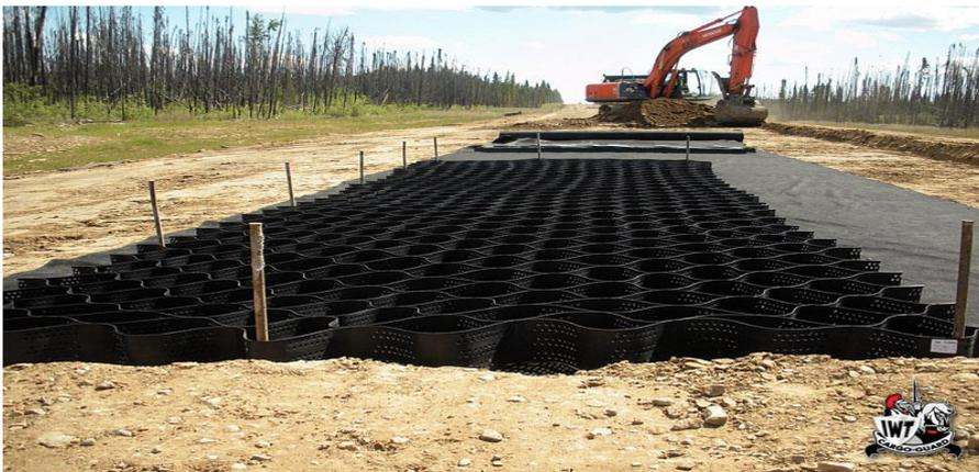
*Figure 1.2 Mechanical Stabilization Using Geosynthetics*
