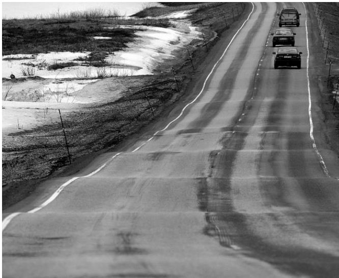
Figure 2.6 The effect of frost heave on roads.
