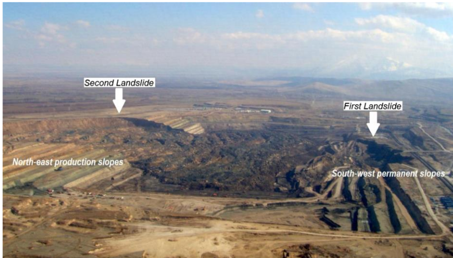
Figure 2.10 Landslide area after both failures (Ozbay et al. 2015)
