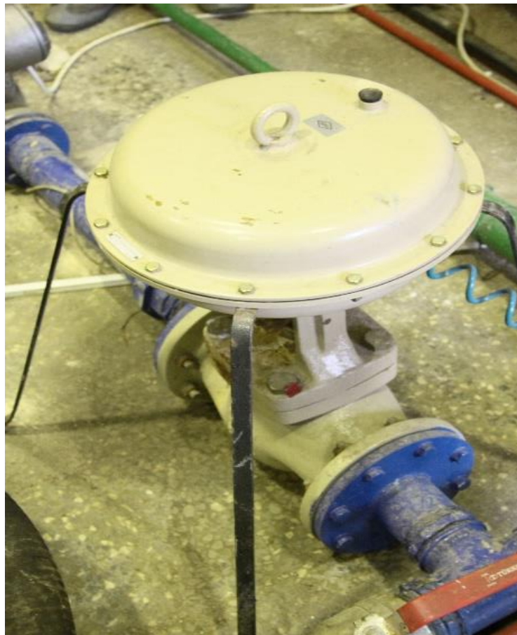
Figure 3. 11 Fisher Pneumatic Control Valve
