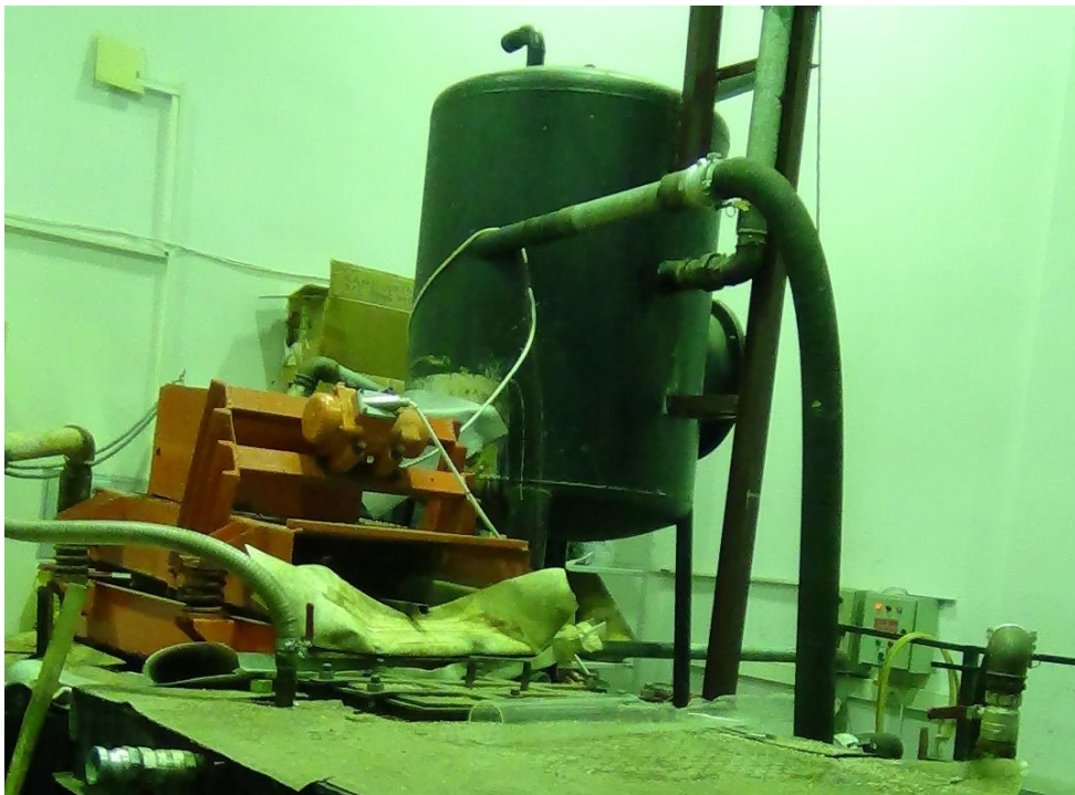
Figure 3. 5 Separation Section and Shale Shaker
