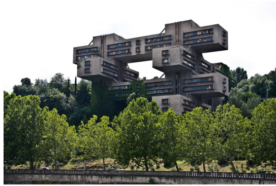
Figure 3.2: Building of Georgia Ministry of Highways ( http://www.architectural-review.com/Pictures/web/c/q/p/Socialist_Modernism_2.jpg )
