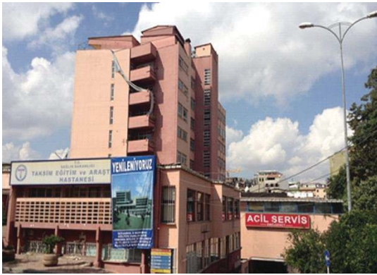
Figure 3.15 Taksim Emergency Hospital before demolishment (Mimari Portal, 2014)
