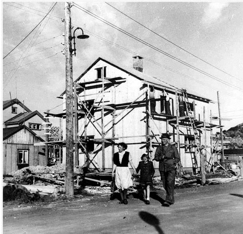
Norway--wooden houses to replace those the Germans destroyed
