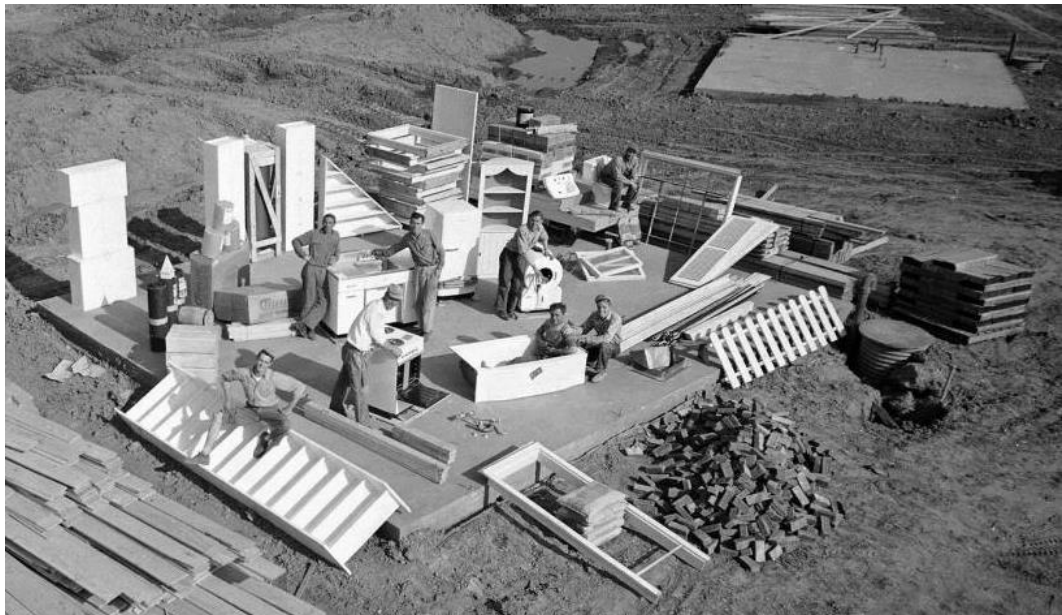
Figure 2.13 Aerial view of construction workers assembling the prefabricated parts of single-family house in Levittown, New York, June 1948.: http://www.gettyimages.com/detail/news-photo/aerial-view-of-construction-workers-as-they-pose-with-the-news-photo/2937859 (accessed June 13, 2015).
