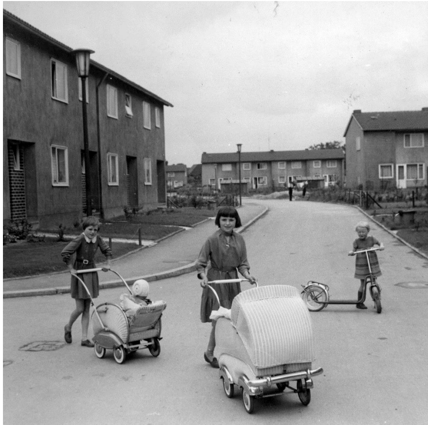
Figure 2.26 A photograph of the everyday life in the neighbourhood of two-storey workers' family houses in the garden suburb of Dortmund-Derne called as MSA-Siedlung.
