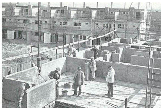
Figure 2.19 Construction of test houses in Frankfurt with prefabricated concrete panels, 1926. Source: https://www.moma.org/interactives/exhibitions/2010/counter_space/the_frankfurt_kitchen#highlights (accessed April 13, 2015).
