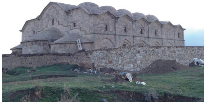
Figure 10. St.Vasilis Church of Misti (Çarıklı) Niğde. The construction of the church was completed in 1922. The Orthodox community of the village could only use it for two years (Karalidis, 2005: 99). It is a giant church for the size of the village community at the time. Photography: Gülen Göktürk.
