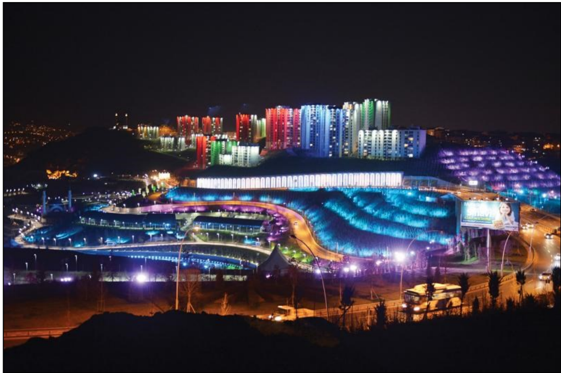
Figure 37. The Lightening of the NEARP
