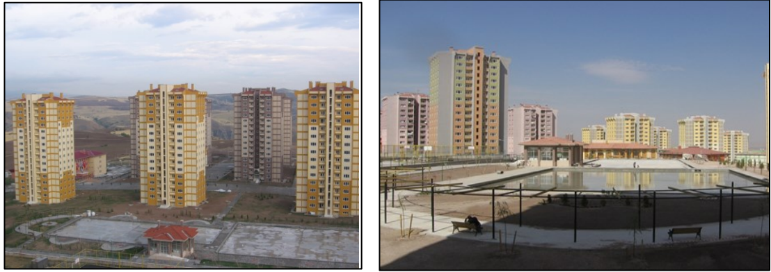
Figure 24. Karacaören Residence Areas
