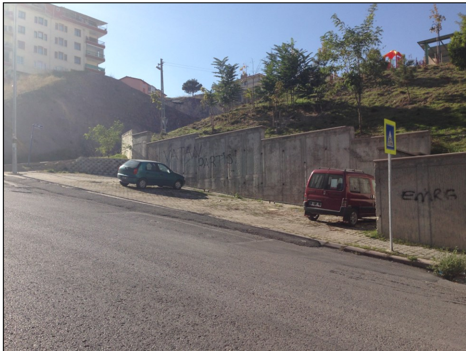
Figure 45. Insufficient Parking Areas throughout the Road
