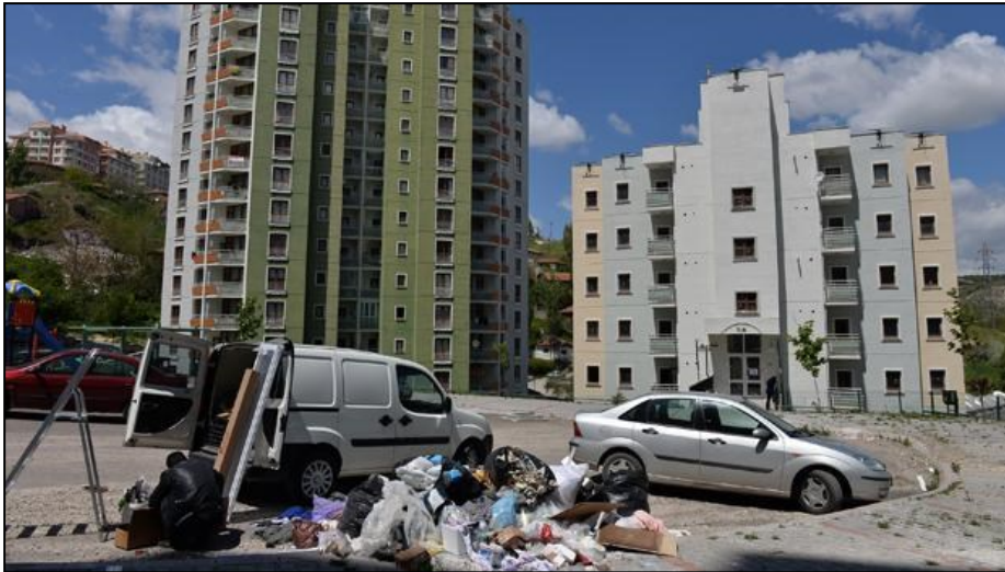
Figure 36. An Example of the Unhealthy Waste Collecting System in the Area
