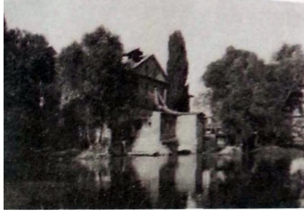
Figure 49: Yasin Çakır Flour Mill (Source: Özaydemir, 2008, p.73)
