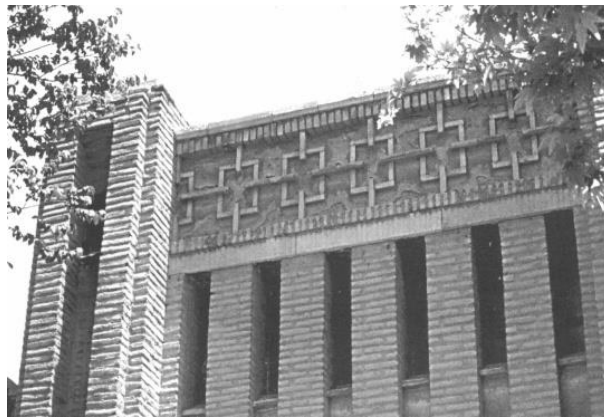
Figure 7: Bricks used as material – Risbaf factory in Isfahan Source: Architecture of First Pahlavi Era. Kiani. P362.
