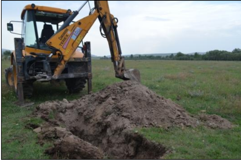
Figure 16. A view during the excavation of the trial pit in the Orta area.
