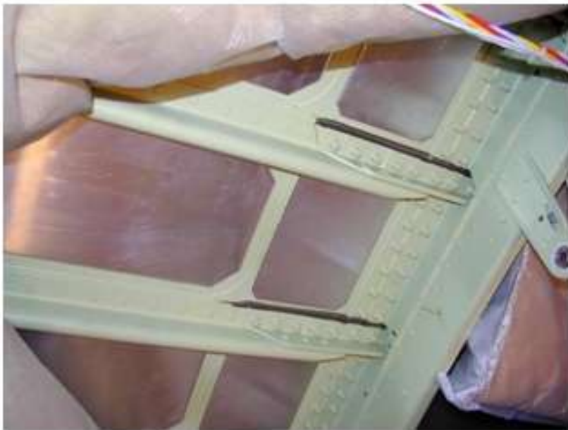
Figure 1-22 Application of damping treatment on aircraft fuselage [57]
