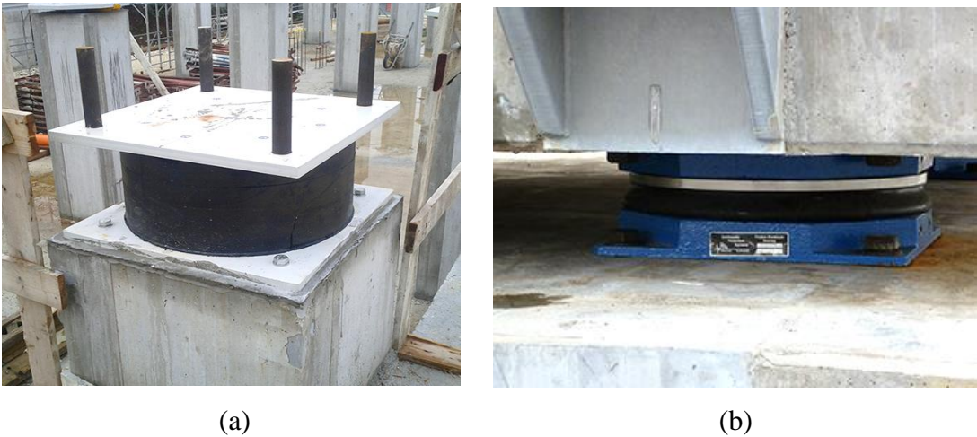
Figure 2.2 (a) Elastomeric and (b) Sliding isolators
