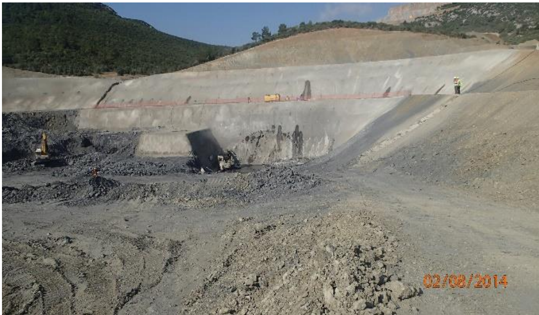
Figure 7. 8 A view of the supported forehead slope at the tunnel entrance.
