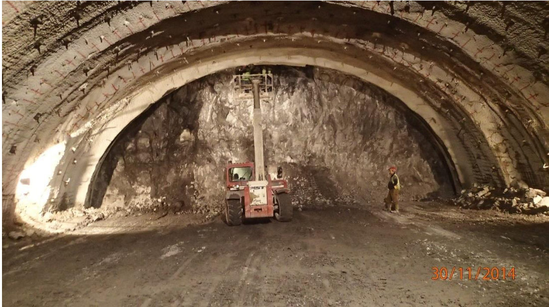
Figure 7. 29 Steel sets installation at Belkahve Tunnel
