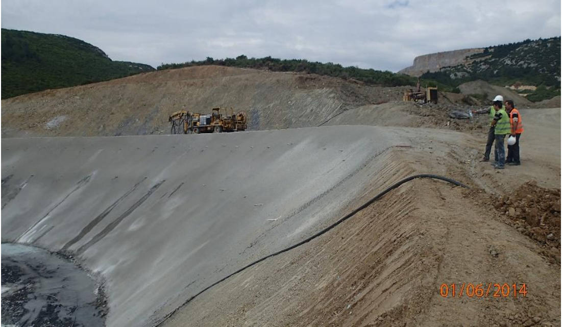
Figure 7. 4 shotcrete and water pipes installed for side slope
