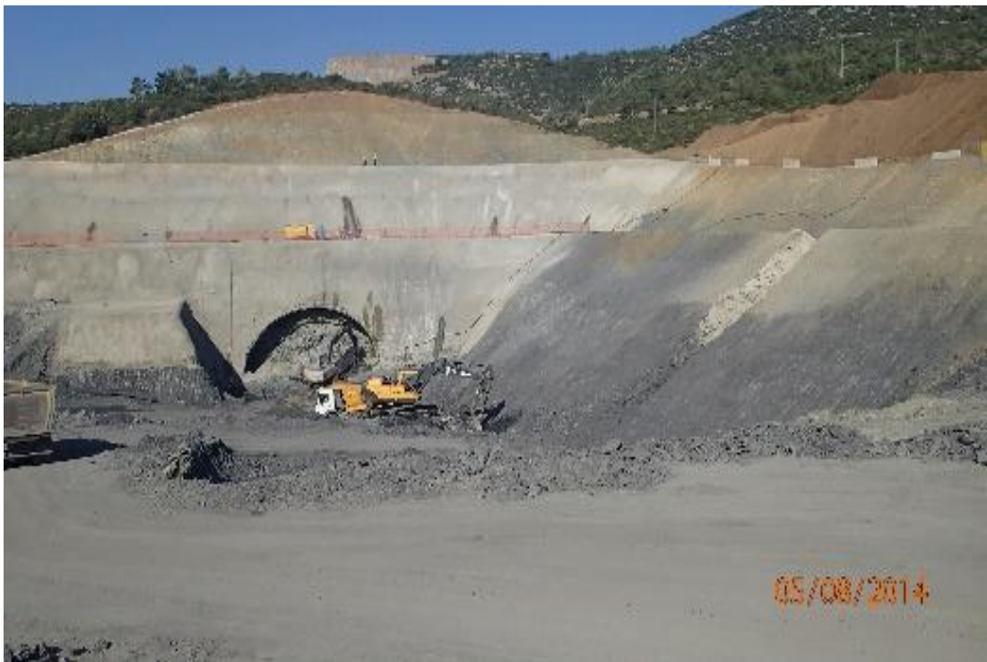
Figure 7. 18 A general view of the excavation at the Belkahve tunnel entrance
