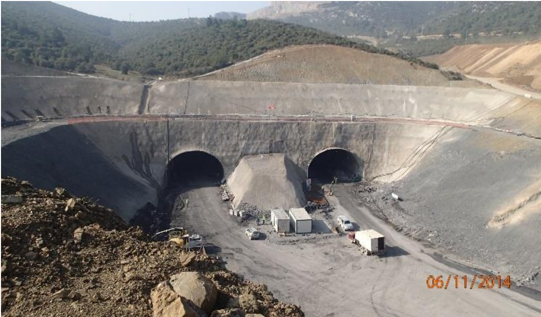
Figure 7. 10 A general view of the supported slopes at the tunnel entrance.
