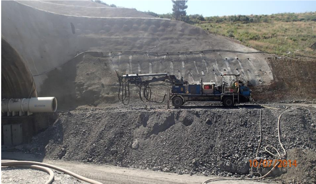
Figure 7. 5 wire mesh and shotcrete installation for side slope
