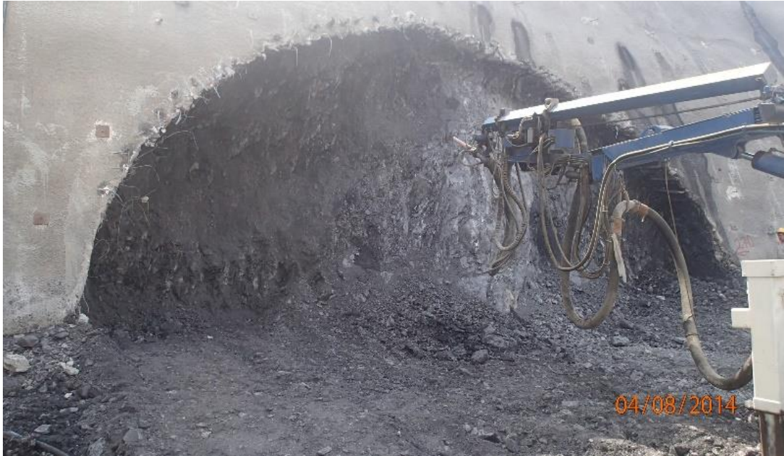
Figure 7. 17 A close-up view of the excavation at the Belkahve tunnel entrance
