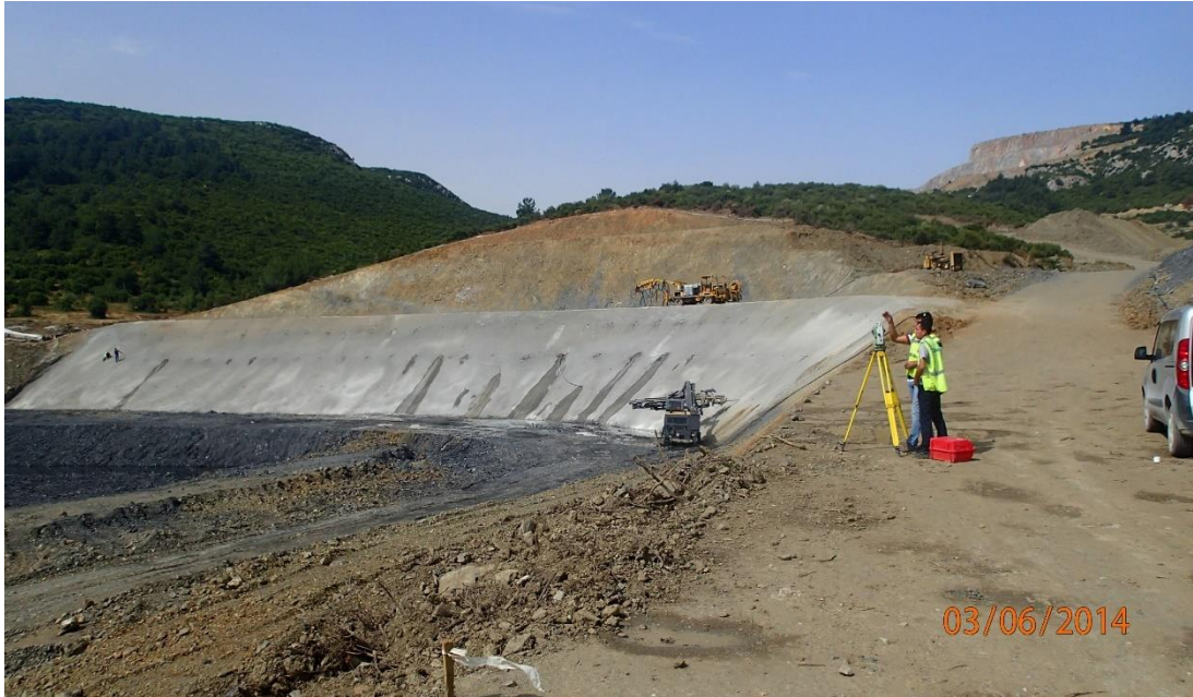
Figure 7. 51 Part of the forehead slope after the supports are installed
