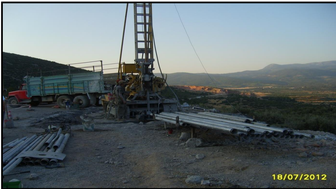
Figure 3. 3 Drilling machine at the middle section of the tunnel route.
