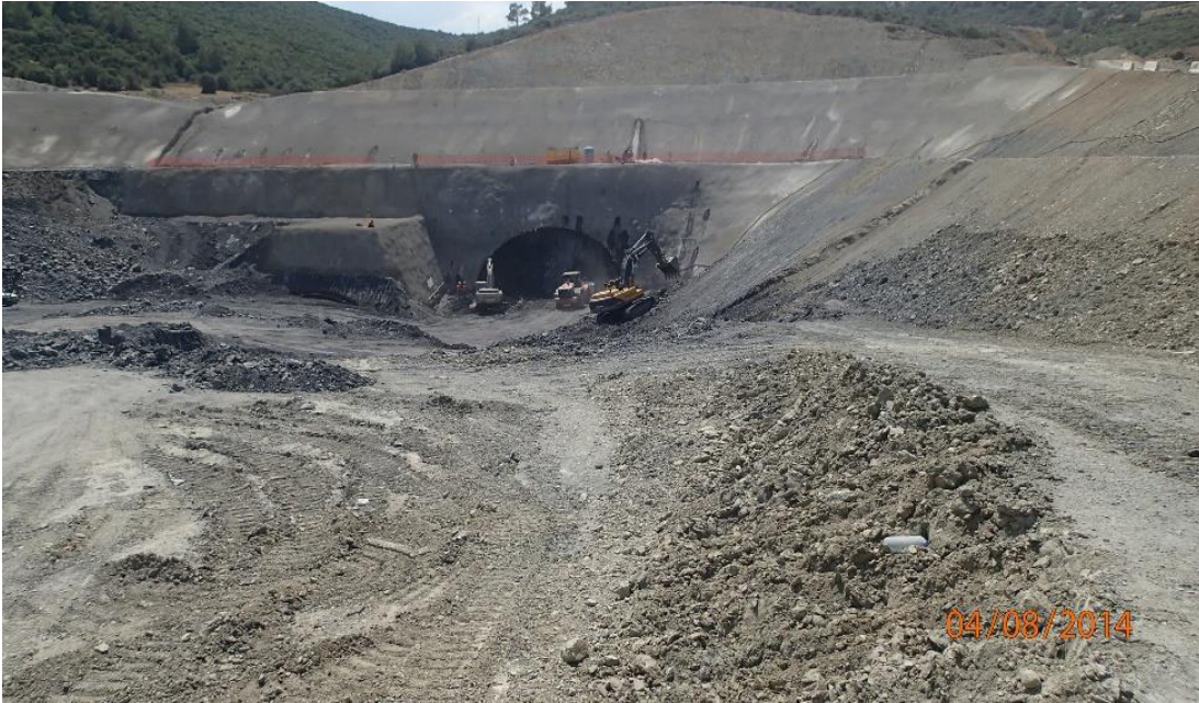
Figure 7. 9 Another view of the supported forehead slope at the tunnel entrance.
