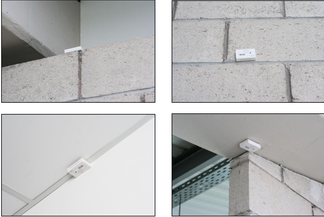
Figure 32: Placement of BLE Tags on Test Bed Environment
