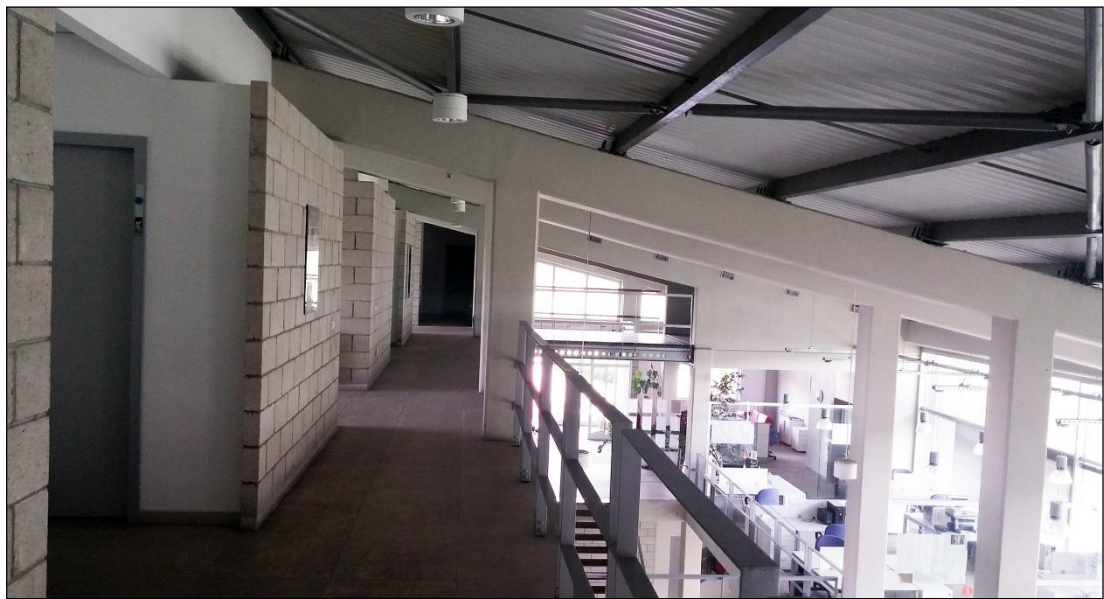
Figure 31: Test Bed Environment - Second Floor of MATPUM Building
