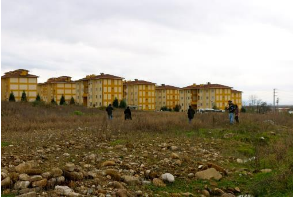
Figure 26 TOKİ mass housing dwelling units located on nearby plot of the project area (Source: Düzce Umut Atölyesi Archive)
