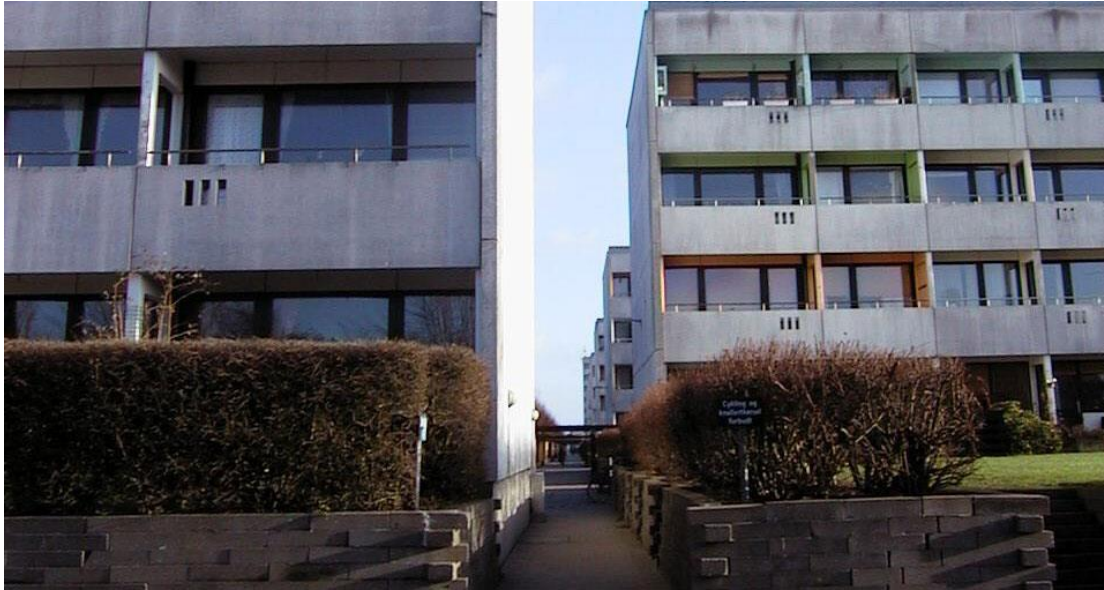
Figure 6-27: Before the renovation. Source: Karen Zwinge Steen/Photoboks
