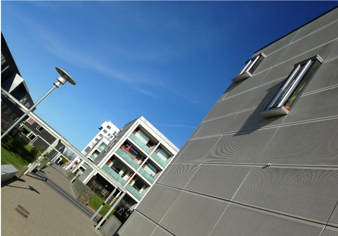
Figure 6-31: Concrete cladding plates on facades to keep authenticity. Bay windows in the narrow facades facing the pergola street. Photo: N. Burak Bican May 2014
