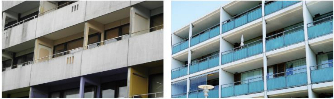
Figure 6-43: Balconies: Before and after. Source: Lejerbo Evaluation Doc. of Gyldenrisparken- 2015
