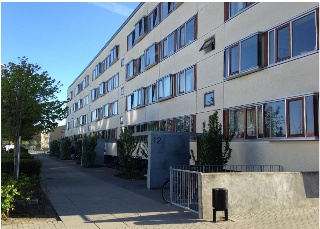
Figure 6-30: Horizontal transparent divisions of facades of housing blocks after renovation.. Source: N. Burak Bican May 2015
