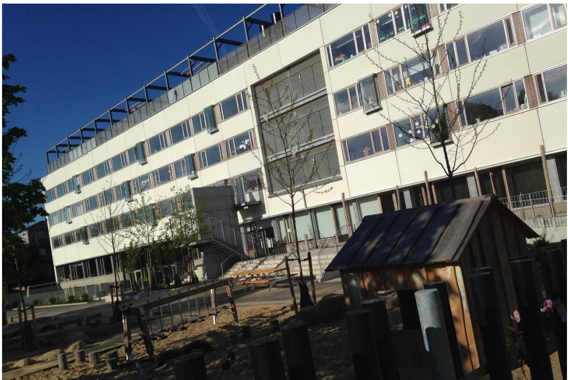
Figure 6-34: The new Children's House after Renovation. FOTO: N. Burak Bican, May 2014
