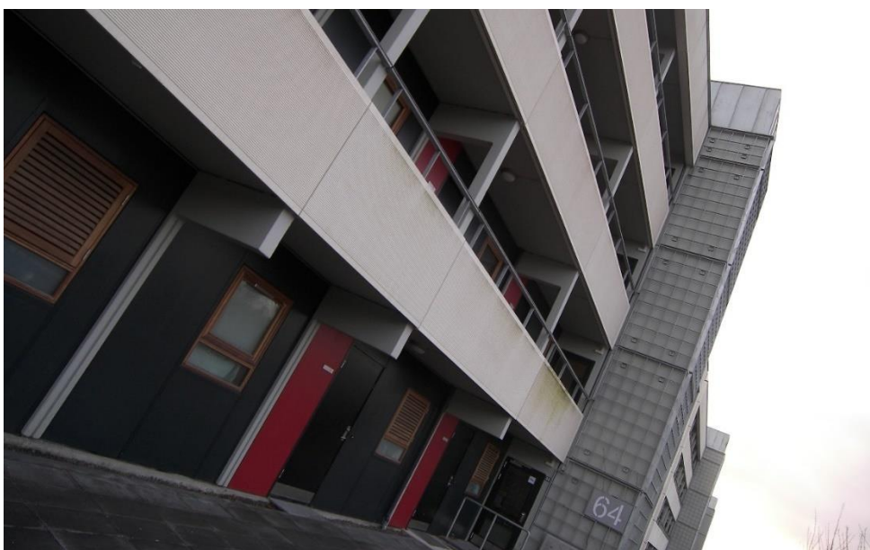
Figure 6-48: Elevator shafts to public balconies. Store Krog. Photo: N.Burak Bican, 12. 2013
