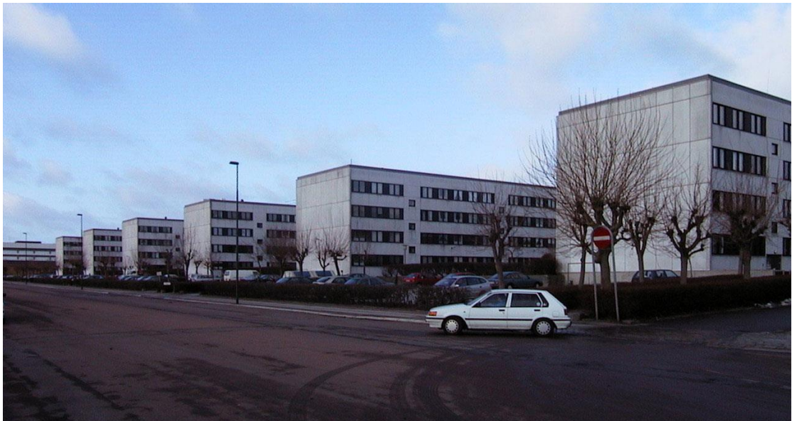
Figure 6-26: Before the renovation. Source: Karen Zwinge Steen/Photoboks
