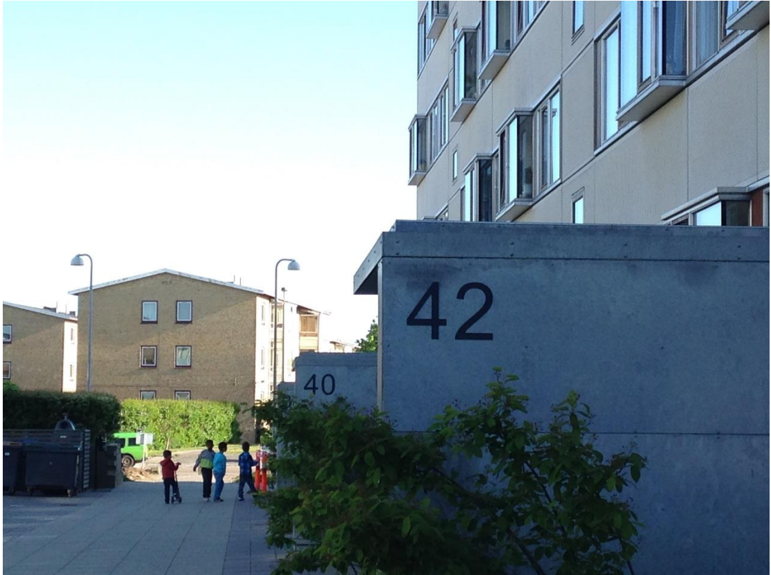
Figure 6-33: Building entrances: to be easily identified. Photo: N. Burak Bican May 2014
