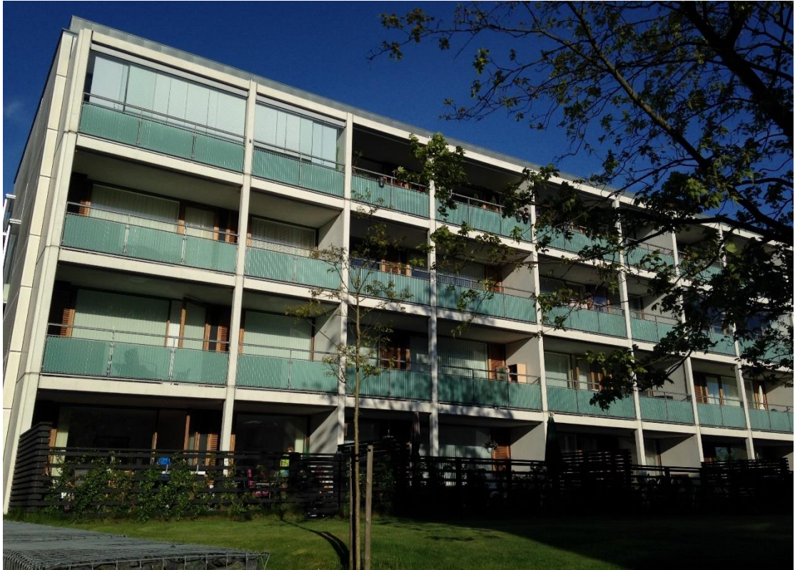
Figure 6-29: A renovated housing block: the facade with balconies. Source: N.Burak Bican, May 2014
