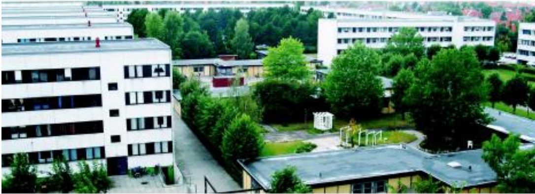
Figure 6-9: Gyldenrisparken: Buildings and common areas before the renovation. Source: KUBEN-LEJERBO Evaluation Material
