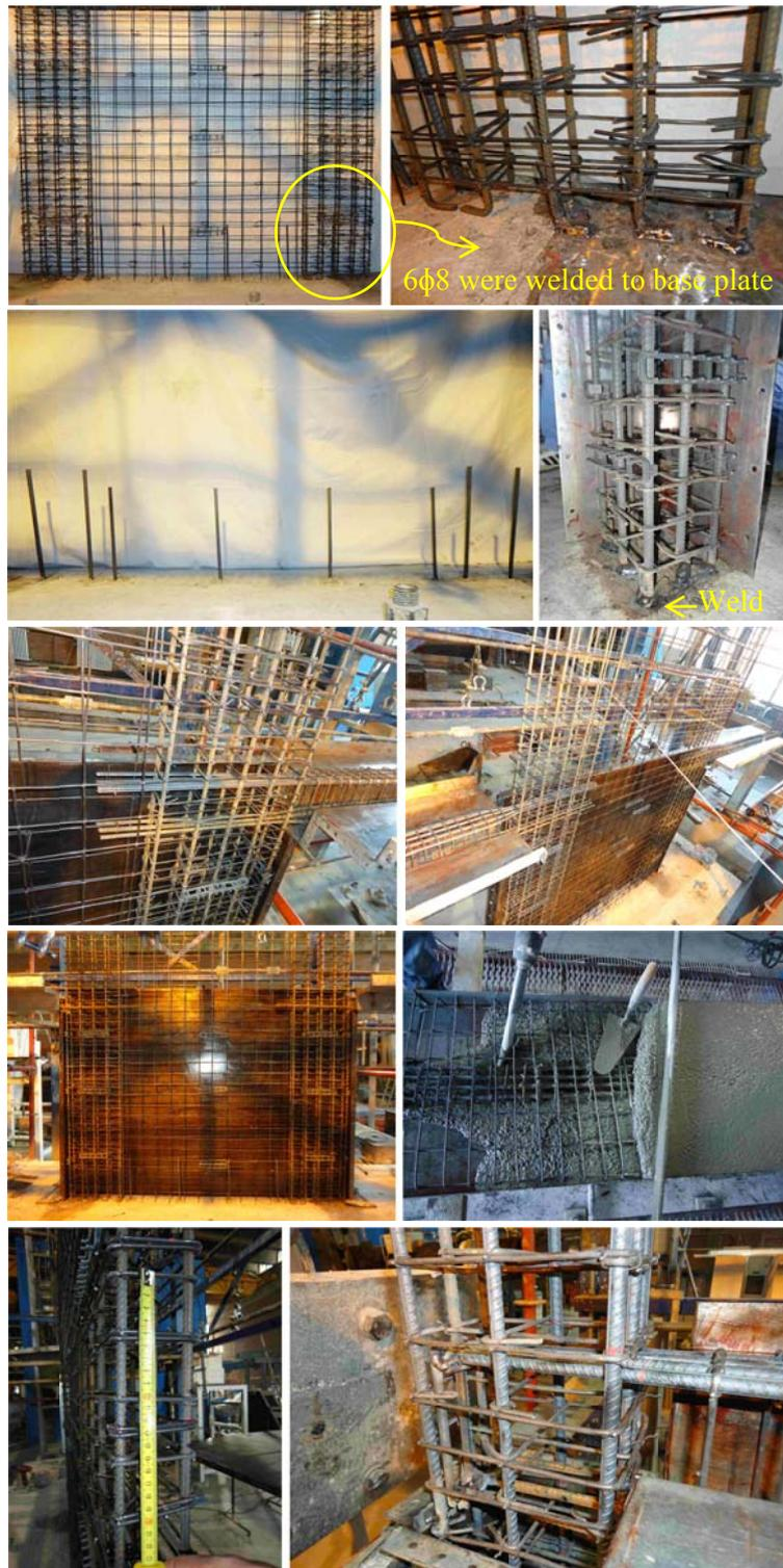
Figure 3.13 Construction stages of RC-SW1
