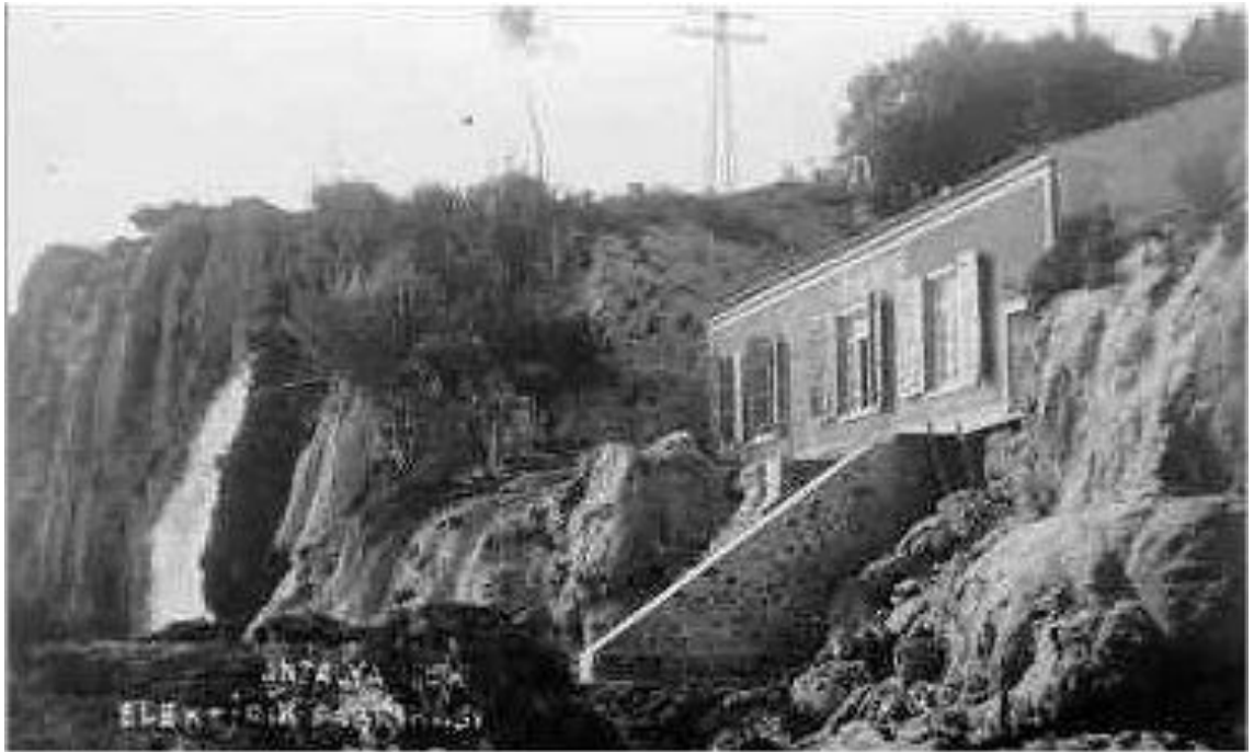
Figure 34 Energy Power Plant (source: Antalya KUDEB)
