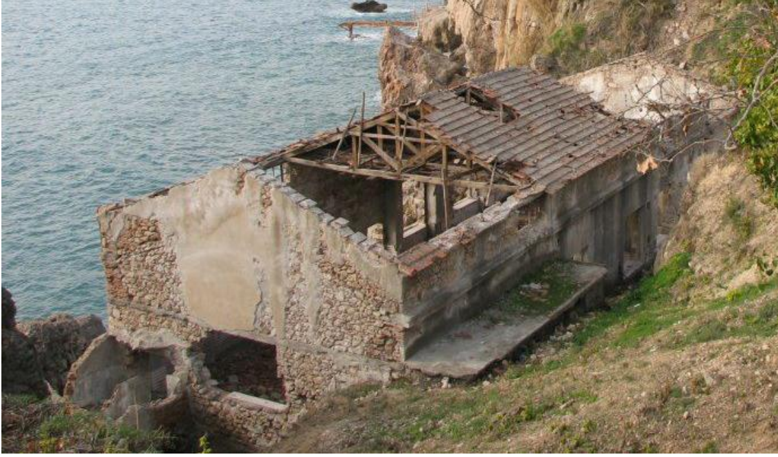
Figure 35 Energy Power Plant (source: Antalya KUDEB)
