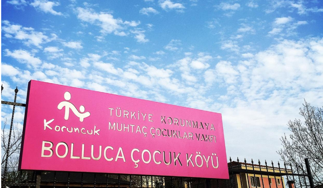
Figure 4.24. The entrance to the Children's Village in Bolluca, Istanbul
