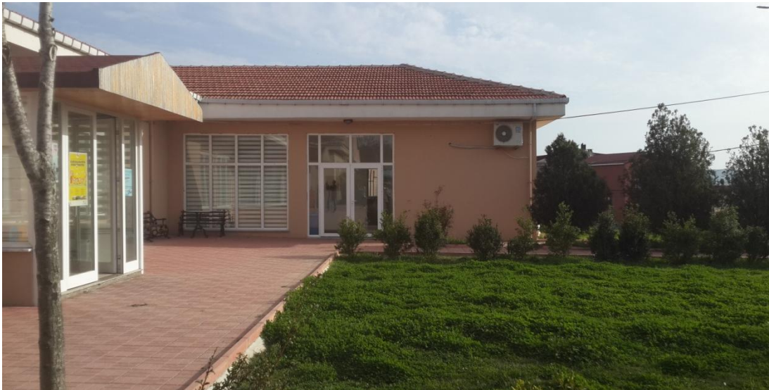
Figure 4.25. The Administrative Building in Bolluca
