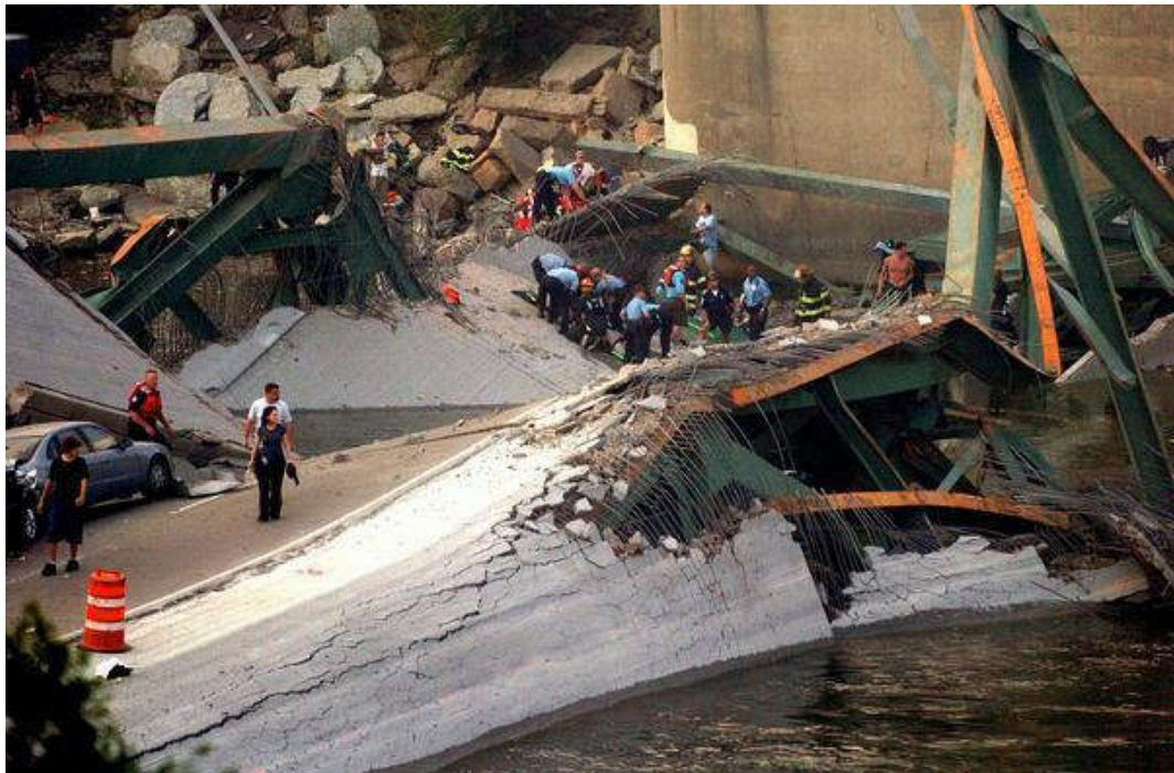
Figure 2.1 Total Collapse of a Bridge in Minnesota (The Denver Post, 2007)
