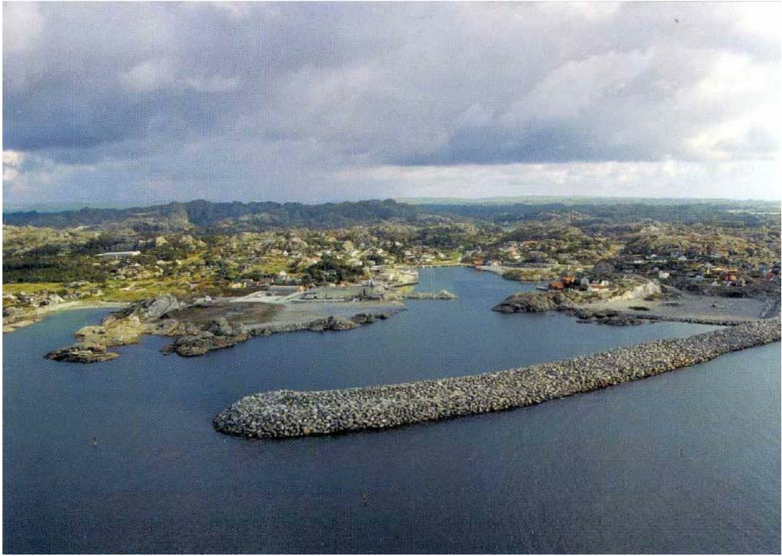
Figure 2.1: Sirevag berm breakwater in Norway.
