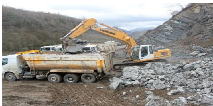
Figure 4.42 Loading of stones, Retrieved from İbrahim Ahmetoğlu, Project Manager of Cengiz Insaat.
