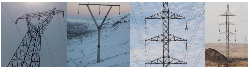
Figure 2.4 Typical suspension (tangent) tower examples (courtesy of Miteng Inc.).
