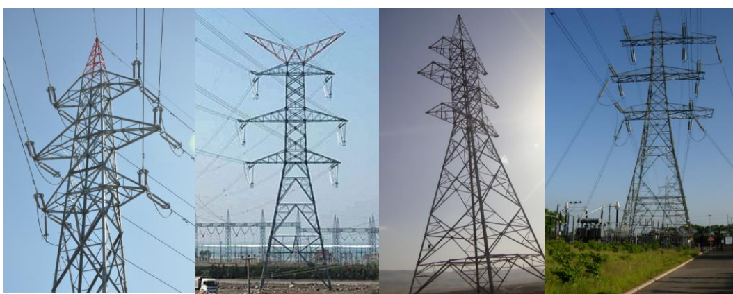
Figure 2.5 Typical angle (tension) tower examples (courtesy of Miteng Inc.).
