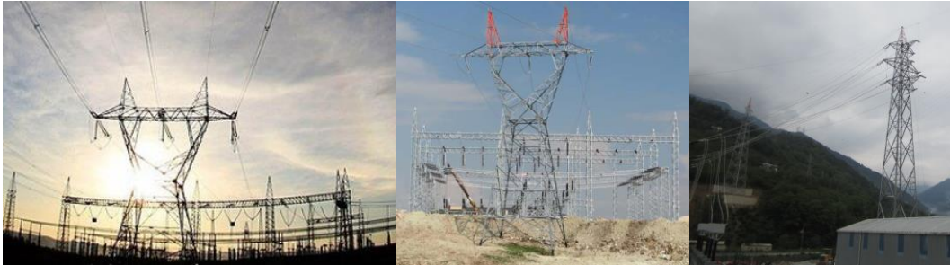
Figure 2.6 Typical terminal (dead-end) tower examples (courtesy of Miteng Inc.).
