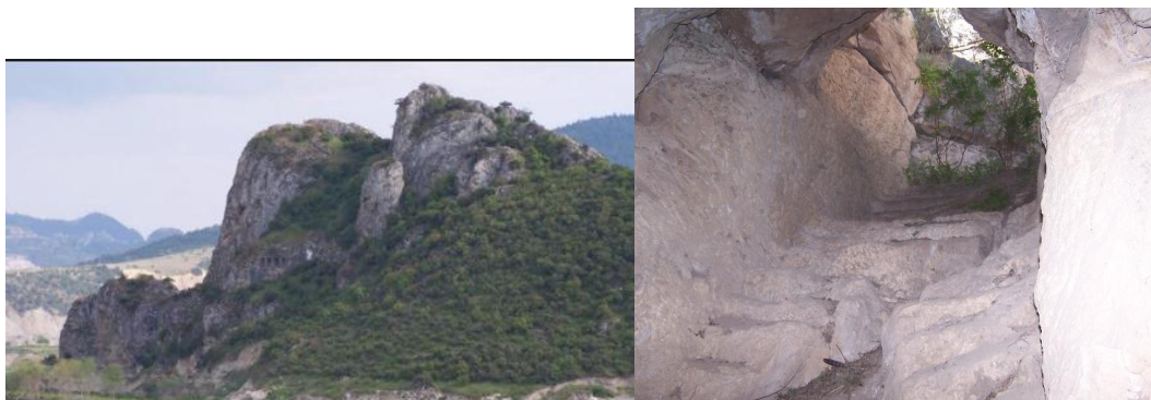
A general view of the fortress and the rock-cut tunnel
