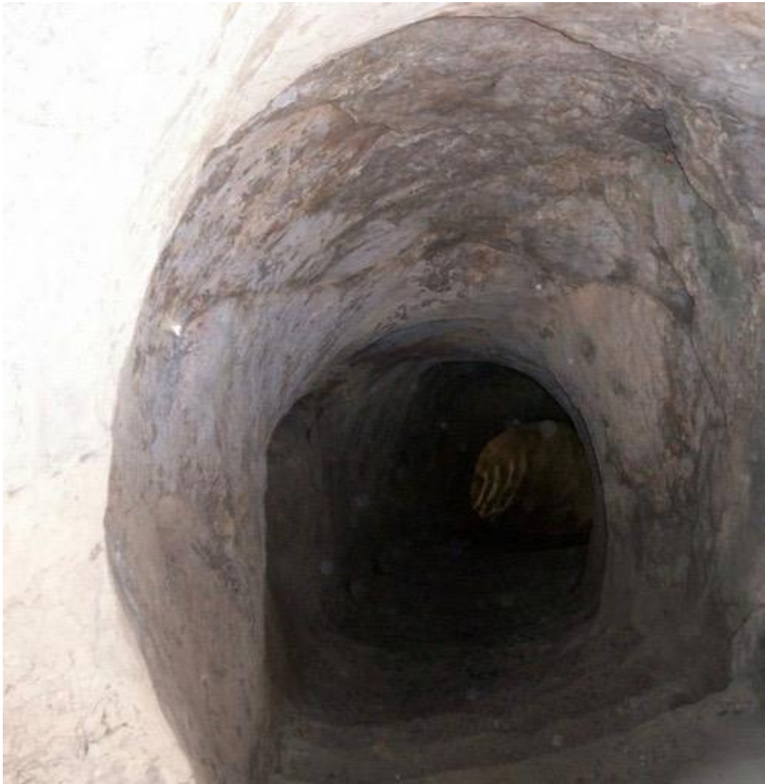
Rock-cut tunnel reach to road (formerly river)
