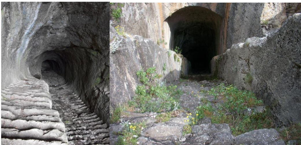
Monumental Rock-cut tunnel
