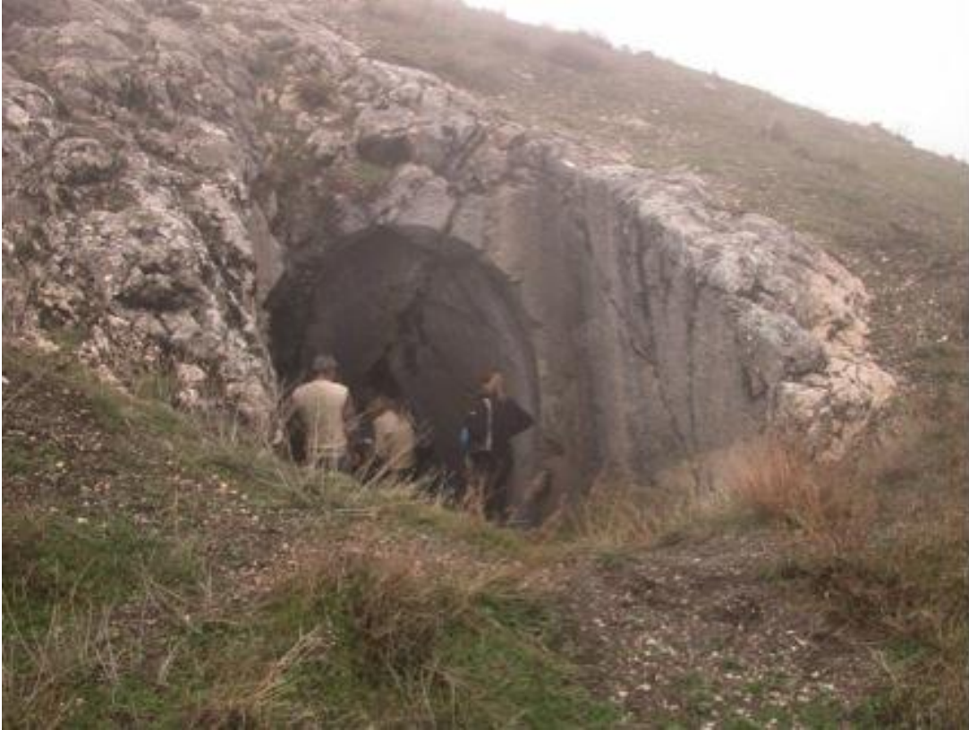
Tunnel Entrance (photo by M. Doğanbaş)
