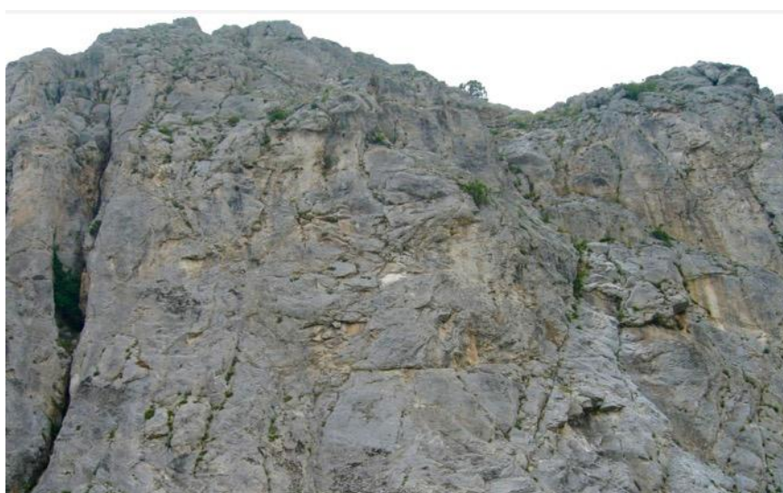
A South face of the fortress
