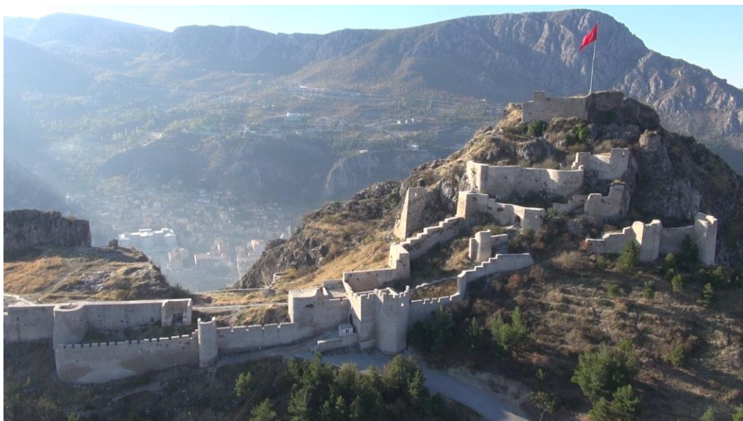
Amaseia Fortress from southwest (photo by PRD Production)
