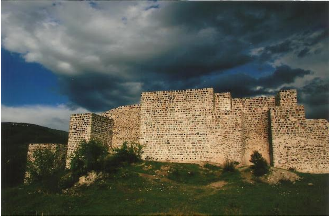
Restored side of the fortress
