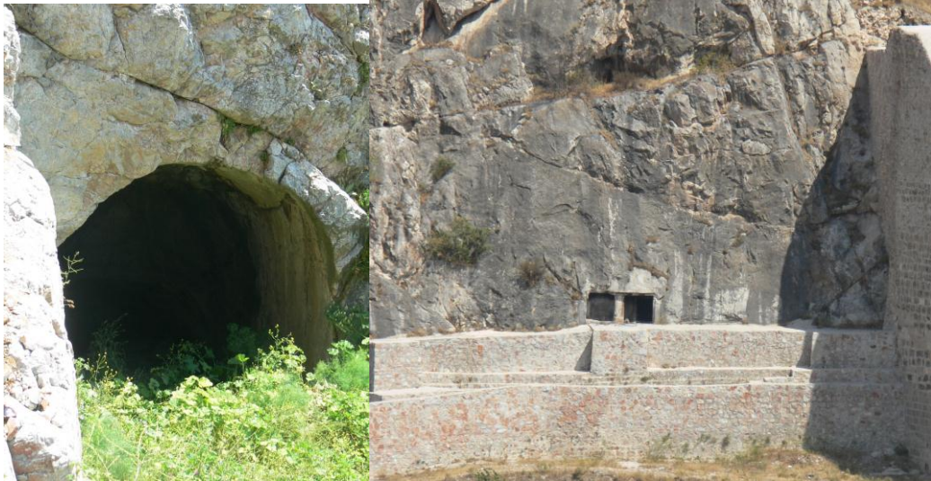
Rock Cut Tunnel on the North side and Rock Cut Tomb on South facade of the fortress
