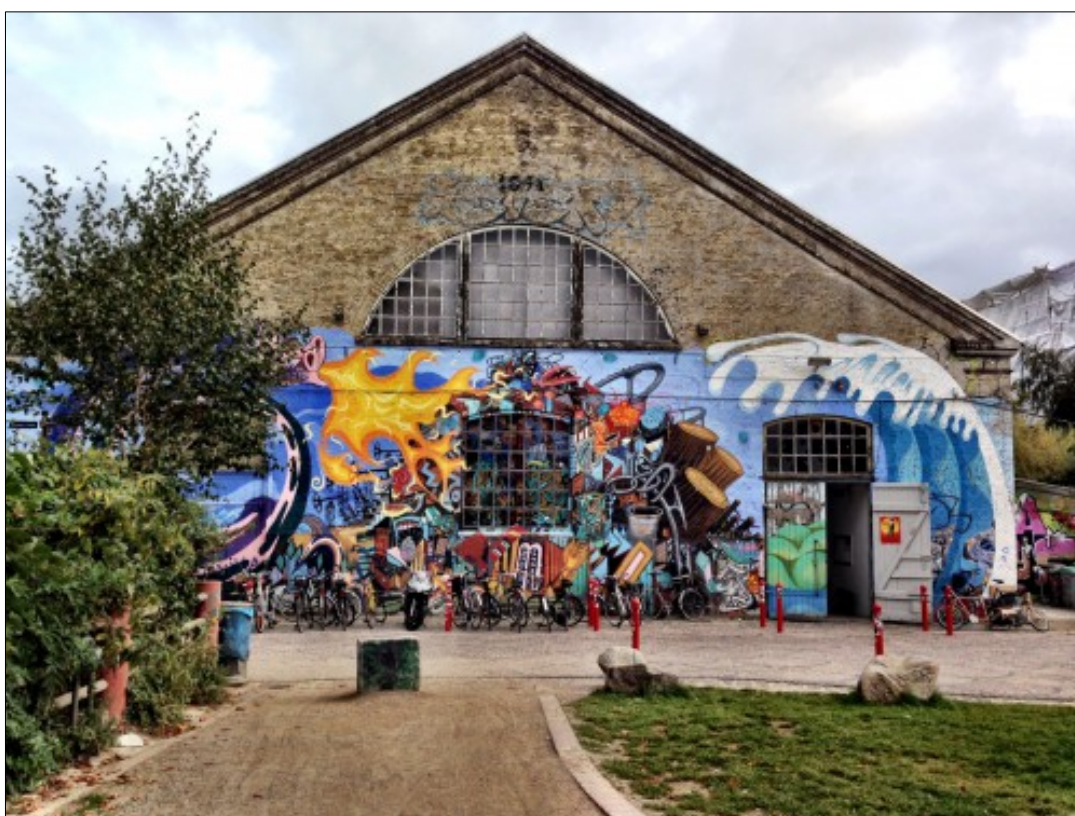
Figure 2.26 One of the old military buildings in Christiania, Copenhagen 27
