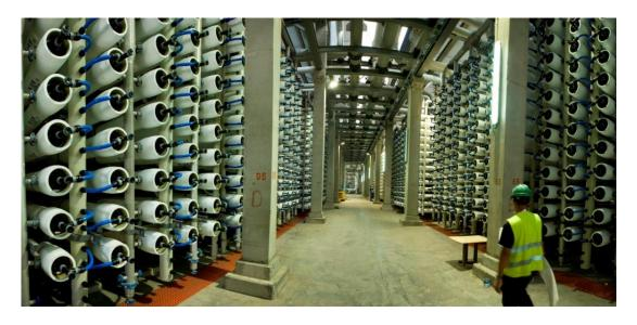
Figure 35: Desalination RO plant in Israel. Stacks can be seen on both sides (Picow, 2010)
