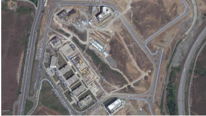
Figure 46: Current construction status of Teknopark İstanbul (retrieved on 01.11.2016)
