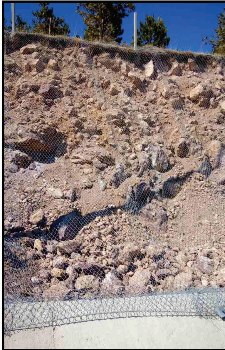
Figure 2.11 Wire mesh protection over the slope on Kayseri-Develi highway.
