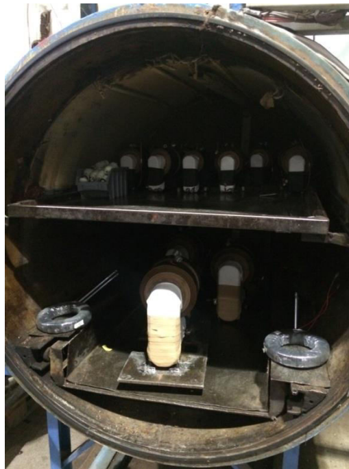
Figure 2-6 Transformer coils under heat treatment
