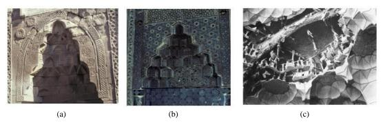
Figure 67. Three ways of Muqarnas constructionCorbeled (a), Superimposed (b), Suspended (c)Source: Hamekasi, Samavati and Nasri. 2011, p.131.
