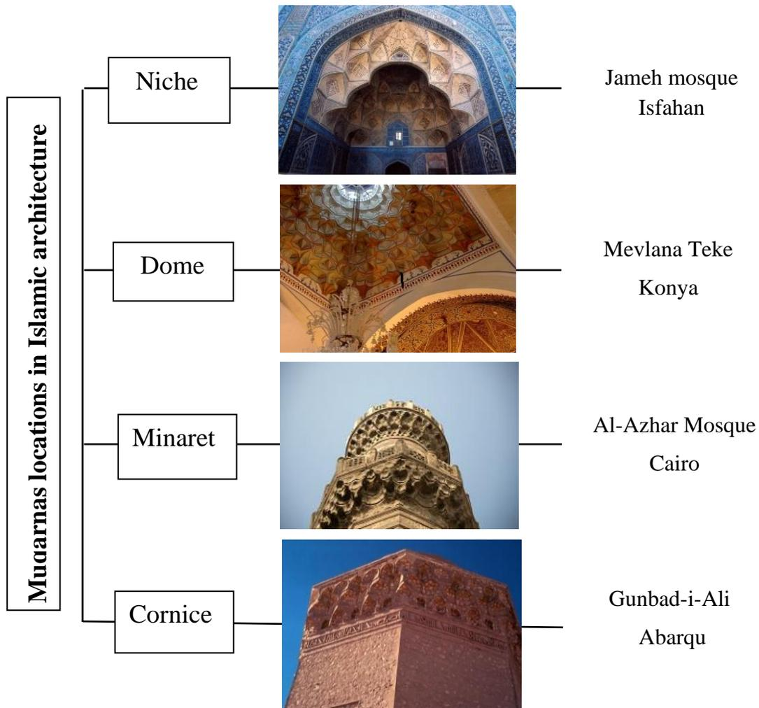
Figure 28. Placement of Muqarnas in Islamic architecture
