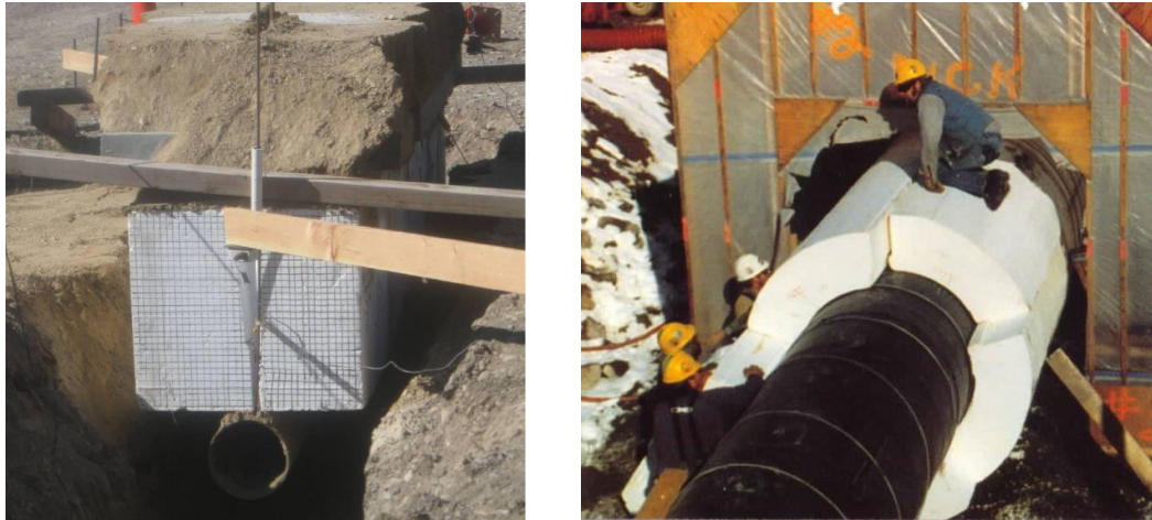
Figure 2.17. Geofabric application for earthquake-induced excess pipe displacement
