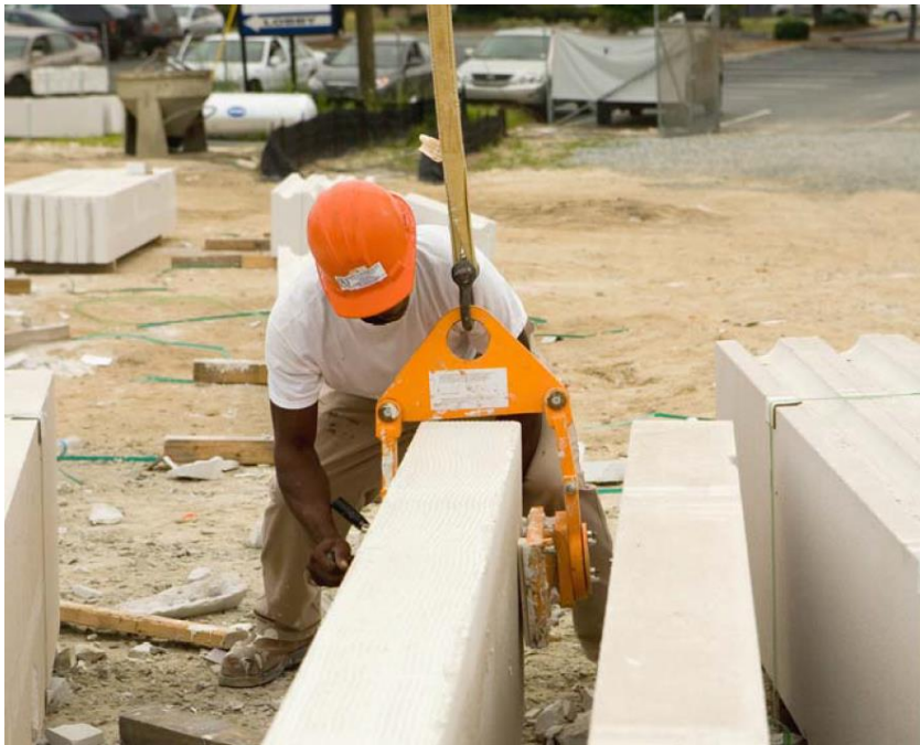
Figure 1.11: Lifting of AAC Panel (Xella, 2010)
