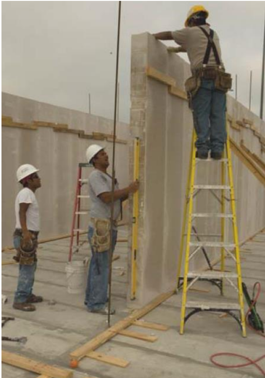
Figure 1.12: Placement of Panel with a Level (Xella, 2010)
