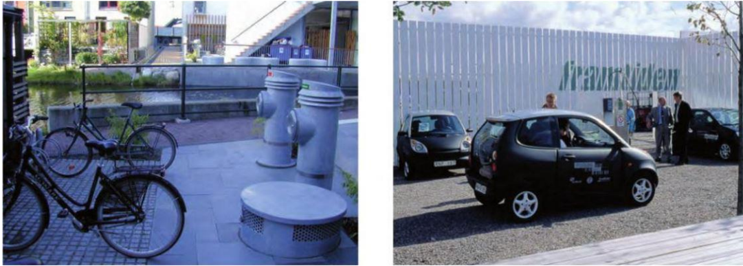
Figure 4. 4. Separation of waste using vacuum refuse chutes and environmentally friendly low emission vehicles. (Ritchie and Thomas, 2013)
