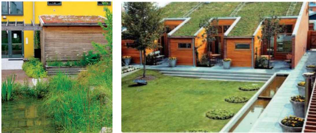
Figure 4. 2. Storm water pond in a courtyard built with regional wetland plants, and green roofs.(Kruuse, 2011)
