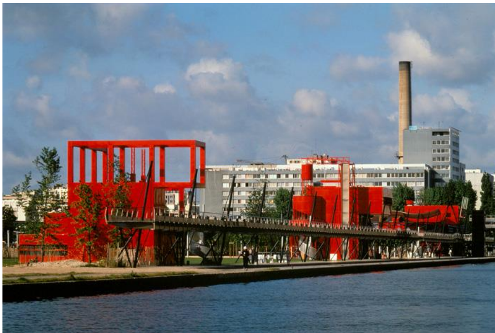
Figure 16: View from point elements in Parc de la Villette (Source: Bernard Tschumi Architects, 1982)
