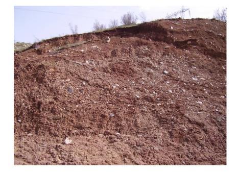
Figure 3.19 The clayey deposits on an unstable cut on landslide zone near Şebinkarahisar
