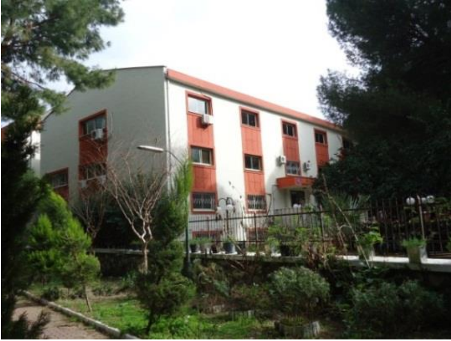
Figure 2. 44. The building after restoration project, (2012)
