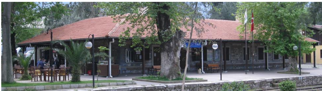
Figure 2. 3 Tire Railway Station and park
