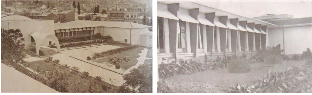
Figure 2. 43. (a)“The building of Municipality newly opened”, (Beş Yılda Tire 1950-1955, 1955:13), (b) The elevation of ‘Tire Municipality’, (Beş Yılda Tire 1950-1955 ,1955:13)
