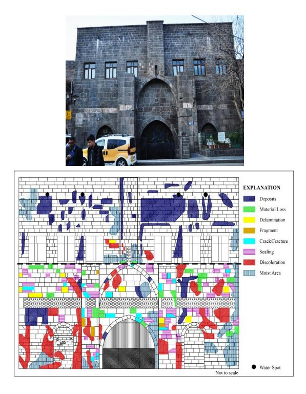
Figure 5.30 The map of visual decay forms on the inner section of the Dağ Gate
