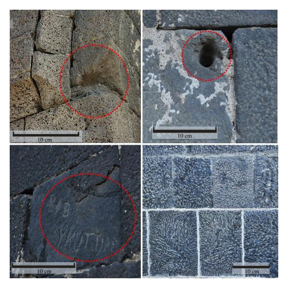
Figure 5.15 Mechanical damages on sections of the DCW (clockwise from top left: impact damage; cavity; scratch/engrave; keying) (damages are indicated by dashed circles)
