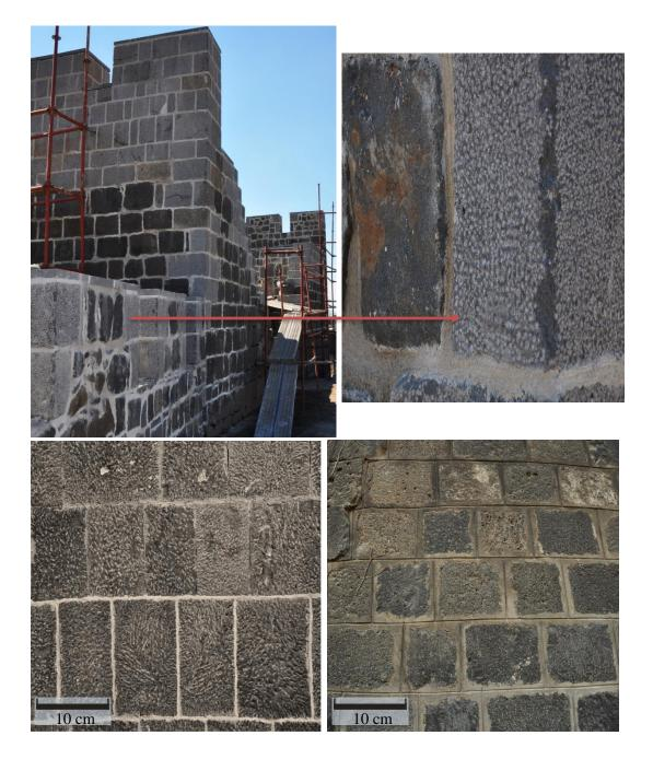
Figure 7.1 Different surface finishes on the DCW
