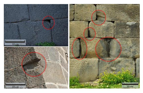
Figure 5.9 Chipping on sections of the DCW (chipping is indicated by dashed circles)
