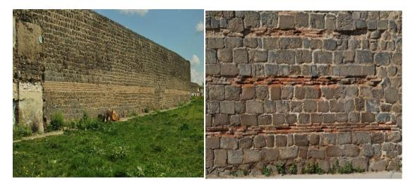
Figure 1.9 Opus listatum (east section of the DCW)
