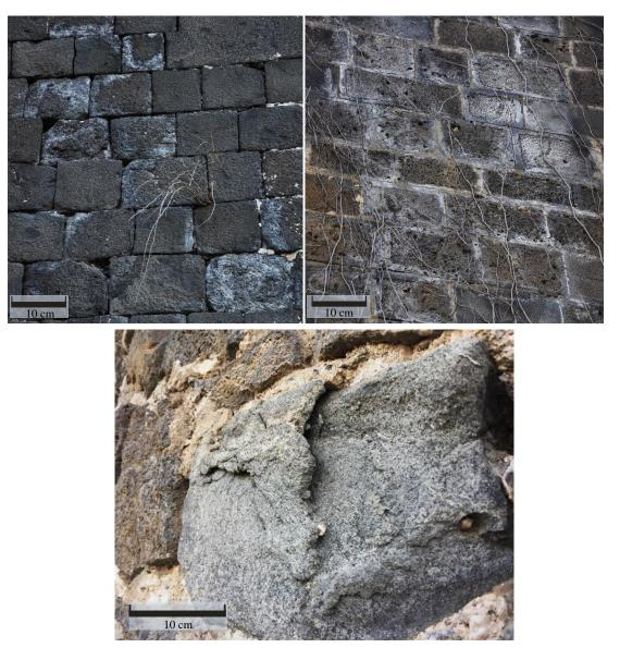
Figure 5.24 Efflorescence patterns on the DCW (the whitish patterns on the stone surface are considered as efflorescence)
