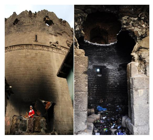
Figure 5.22 Discoloration of the stone surface due to human-induced activities (left: A tandoor located just under the Yedi Kardeş Tower; right: Inside part of an abandoned tower) (left image credit: Aşılı, 2010)
