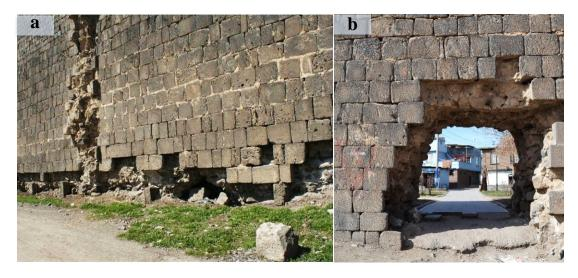
Figure 1.6 Dismantled and breached wall sections (a) Dismantled wall base; (b) A gateway opened by breaching the wall
