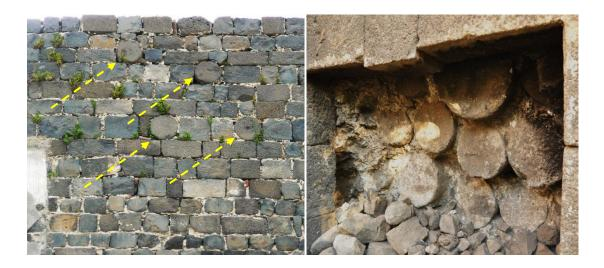
Figure 1.10 Cylindrical basalt applications (south and north section of the DCW)
