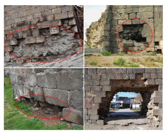
Figure 5.16. Dismantled stone blocks and a breach in the DCW (dismantled sections are indicated by dashed circles)
