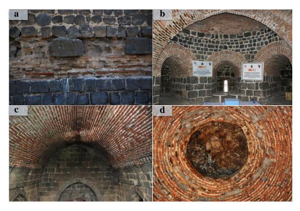
Figure 1.15 Brick applications on different sections of the DCW (a) Brick courses; (b) Brick domes and arches (Melikşah Tower); (c) Brick vault (Melikşah Tower); (d) Brick dome (Keçi Tower)
