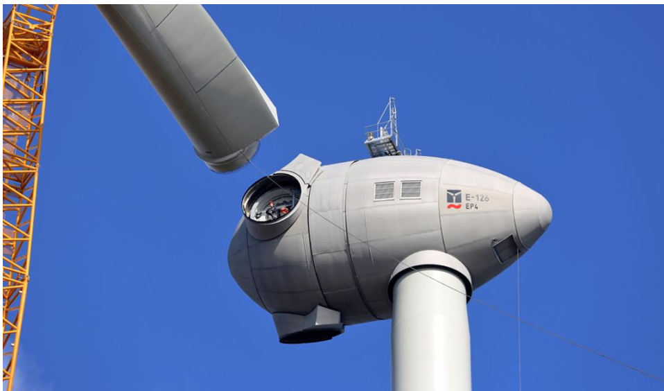
Fig. 2-10. Enercon E-126 EP4, 4.2 MW wind turbine during the installation [44]
