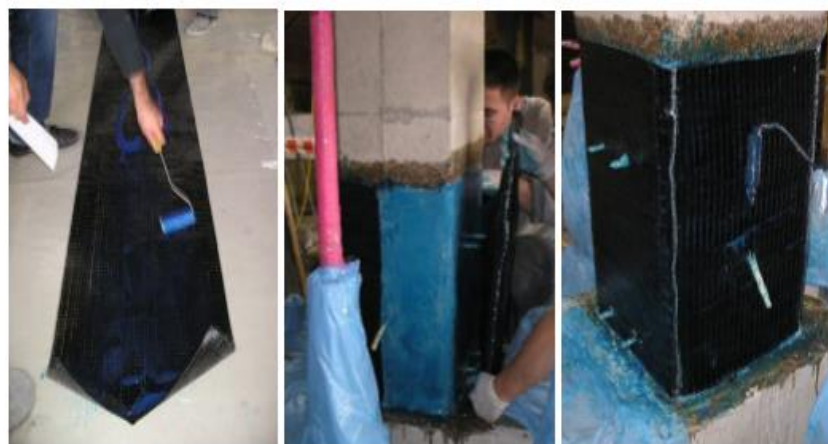
Figure 1.8: Confining of RC columns with CFRP (Ozcan, 2009)
