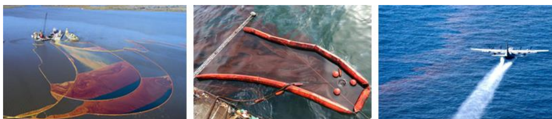
Figure 1.9 Application of booms (left), booms and skimmer (middle) and plane dropping oil-dispersing chemical (right) (NOAA, 2015)
