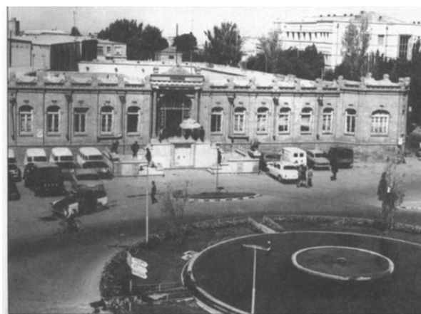
Figure 4.10: The Building of new Police department in Tupkhaneh square Source: URL 8
