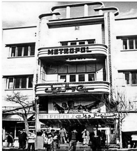
Figure F.1: Cinema Metropol - built in the first years of 1920s Source: URL 22
