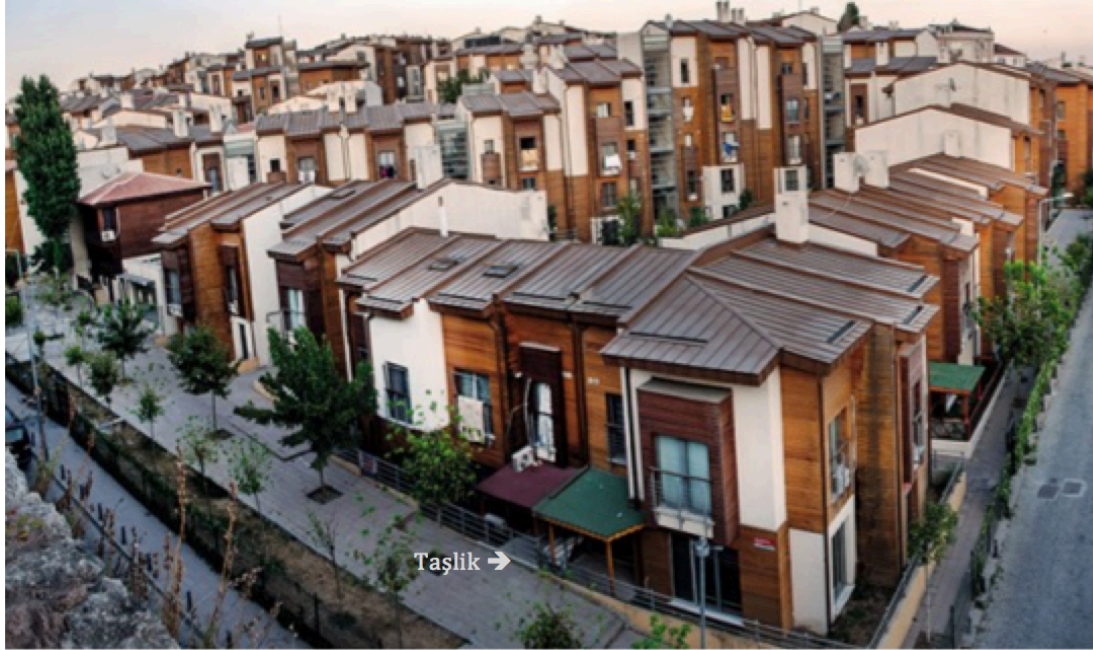
Figure 4-28: Sulukule after regeneration project Source: Google maps (Last accessed:01/03/2018)
