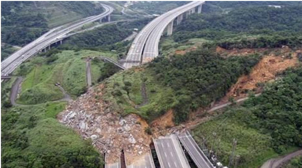
Figure 1 - Taiwan freeway landslide (Taiwan National Freeway Bureau)
