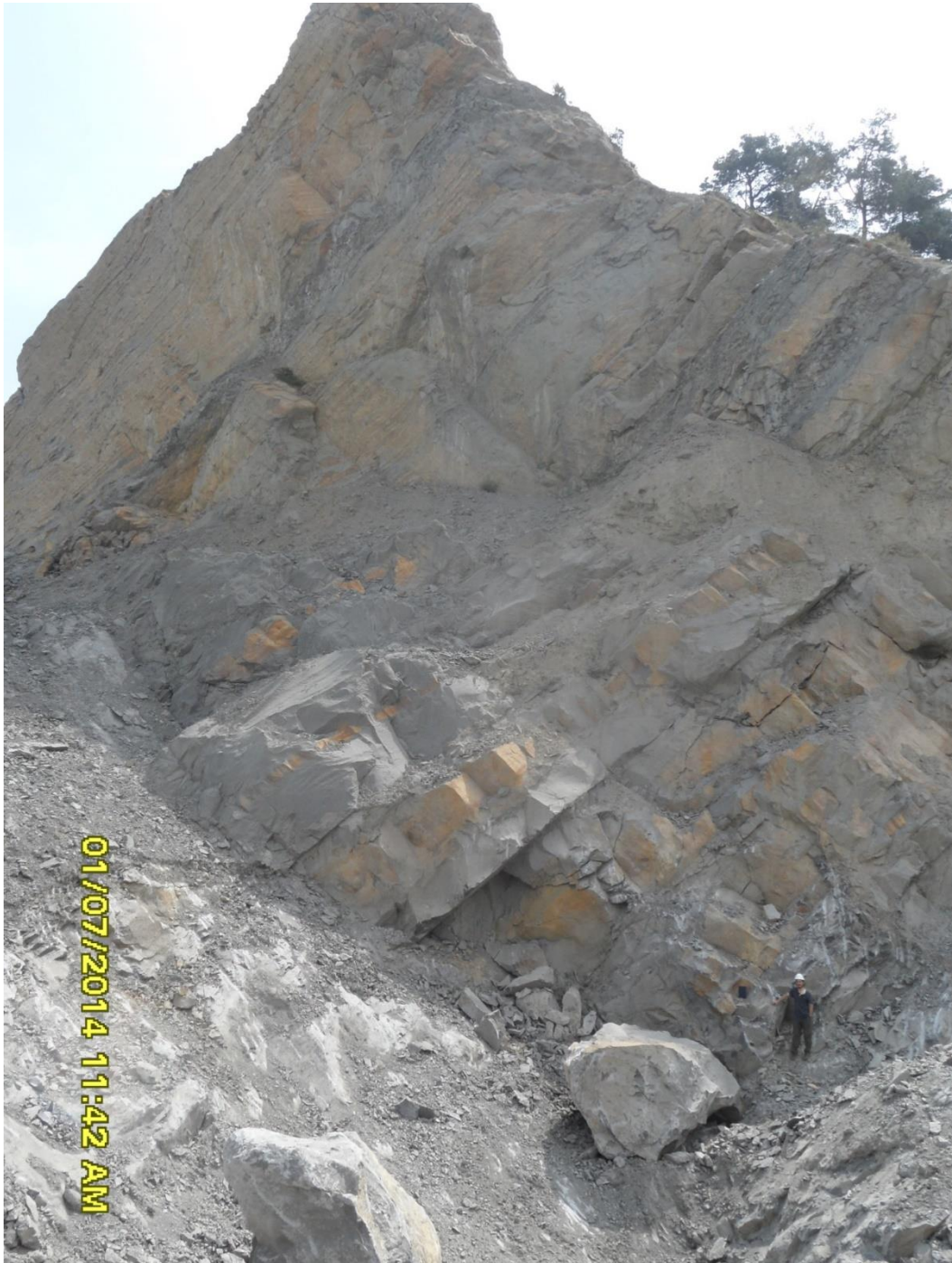
Figure 5. Rock mass structure at Kilimli, Zonguldak No 50 Turkish State Railway Tunnel and slope excavation site
