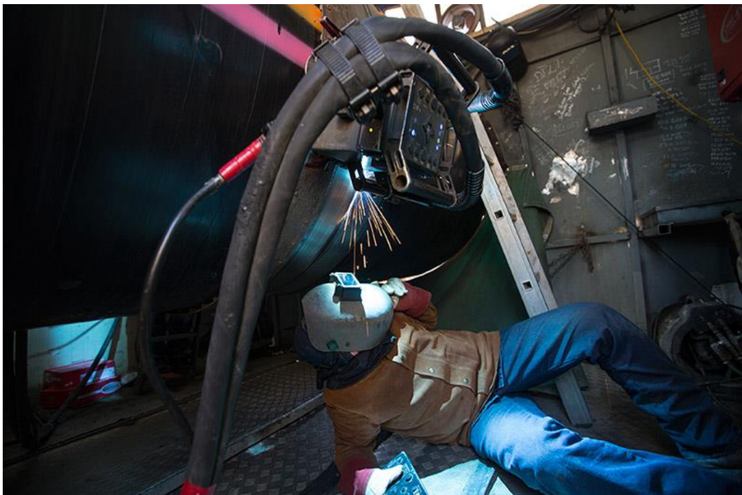
Figure 2. Automatic GMAW on 56" line pipe steel [12]
