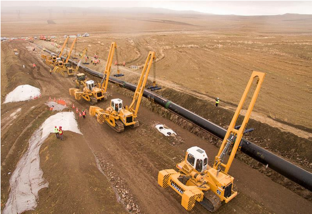
Figure 3. Pipe lowering process applied by side boom tractors [12]
