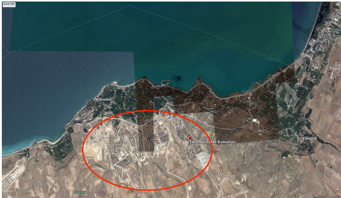
Figure 4.3: Edremit TOKİ Houses & Erdemkent Neighborhood (Source: Google Earth)
