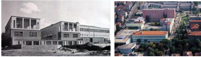
Figure 26 The original building by Ernst Egli, 1938; Ankara University School of Political Sciences after the additions by Tokay and Tayman
