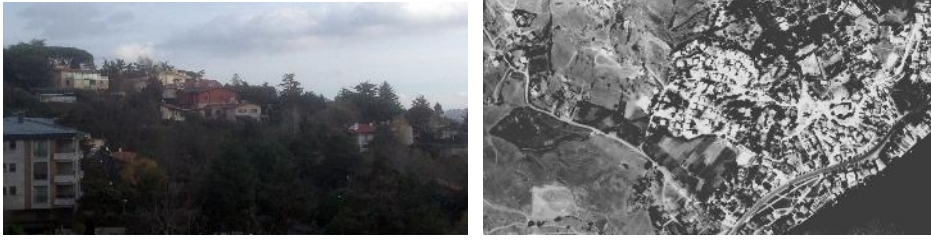
Figure 21 Yeniköy Ankaralılar Cooperative Villas, with Yılmaz Sanlı, 1953-54. View from the southwest and air photograph of 1966.
