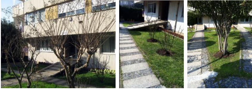
Figure 67 Tayman + Ayhan Apartments, Nispetiye Street, Etiler, 1969.
