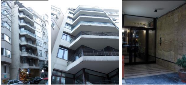
Figure 69 Tayman Apartments, Hüsrev Gerede Street, 1970.
