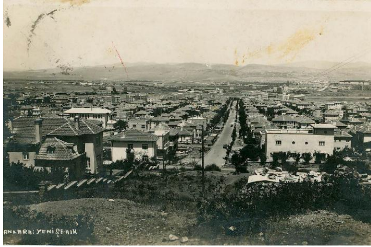
Figure 13 Yenişehir, Mithat Paşa Avenue from Kocatepe, indicating the building stock in 1935-1937 Source: Koç University Vekam Archive
